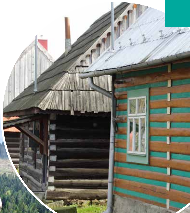
Wooden constructions in Osturňa
